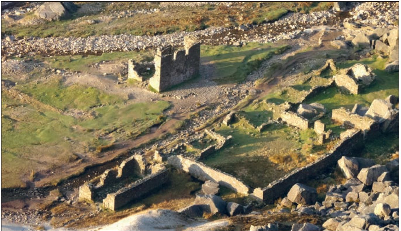
Figure 32. The first rays of the morning sun catch the stonework of the 'Miners' Village', something of a misnomer, as it was not residential, but an industrial complex comprising office, stores, forge and workshops for the mines and the dressing floor. The truncated remains of the Cornish rolls crusher house can be seen in the centre
