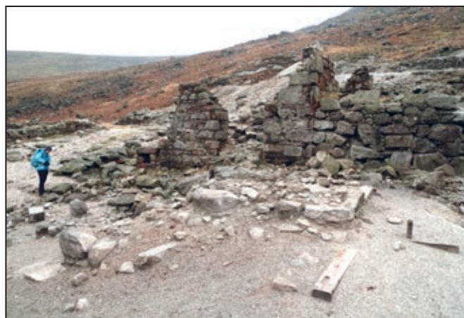
Figure 16. The extant remains of the Cornish rolls crusher house and the emerging stone and framework of a jiggling platform sited in front. The wheelpit is to the far left
