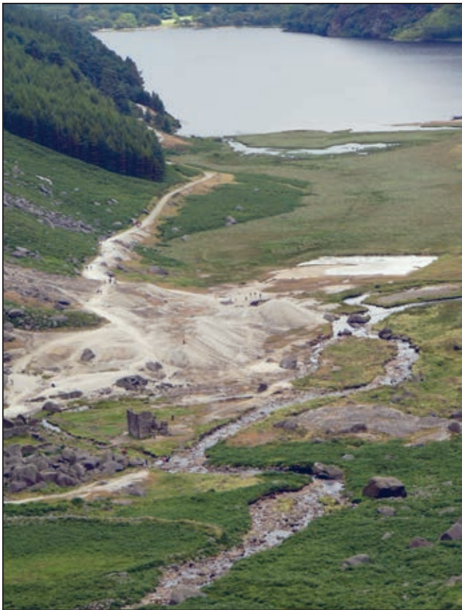
Figure 23. The square outline of the MCI tailings dam (centre right), built to prevent lead contaminating the lake. The halvans dumps are opposite the crusher on the right
