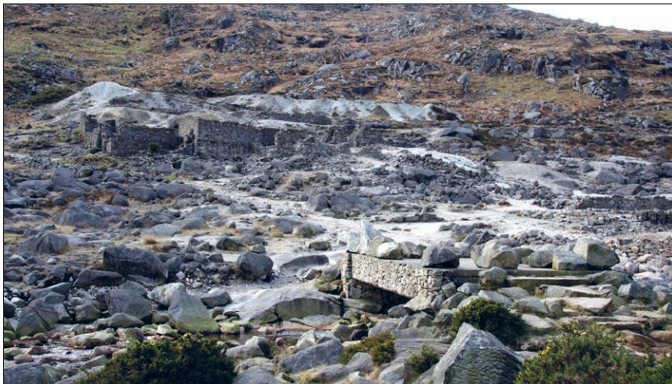
Figure 15. General view of the Hero dressing floor, Glendasan. The grey-white finger dumps of spoil from Old Hero Engine shaft can be seen behind the walled compound known as the mine yard, constructed of granite blocks on top of a massive platform of random moorstone built into the slope of the hill
