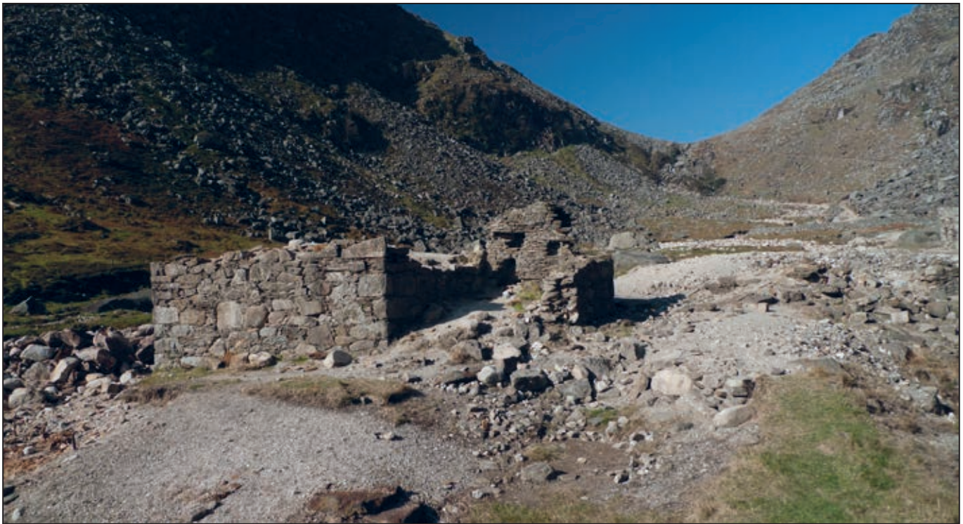
Figure 31. The site of the Cornish stamps, erected in about 1855, contains a unique suite of features which makes this the most important site of its type in Ireland. It is of significant heritage value
