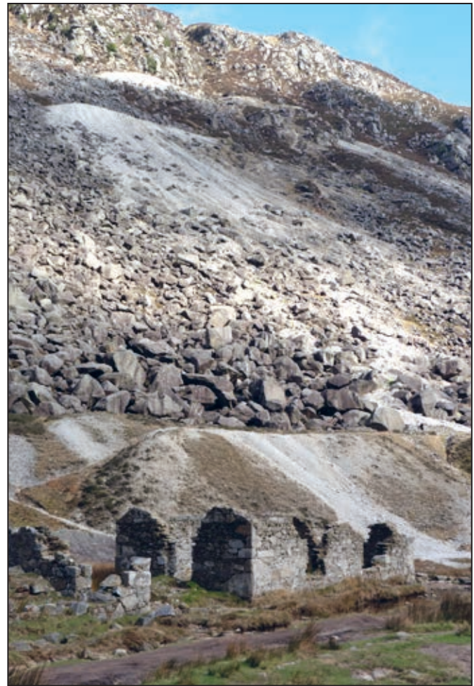
Figure 34. This building (GL-14A), shown on all historic mapping, might have functioned as an ore store, where the lead concentrate was safely secured prior to being weighed, bagged and transported to the Ballycorus Smelting Works
