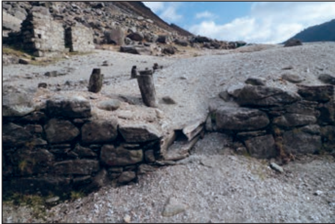
Figure 26. Inclined box launder (centre) emerging through a damaged section of the revetment walling of the primary dressing floor. A set of posts for a tramway to the crusher can be seen centre left and the bouse team far left
