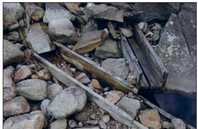
Figure 29. Two wooden launders that conveyed slimes from the tyes and jiggling area in front of the crusher house once crossed over each other
