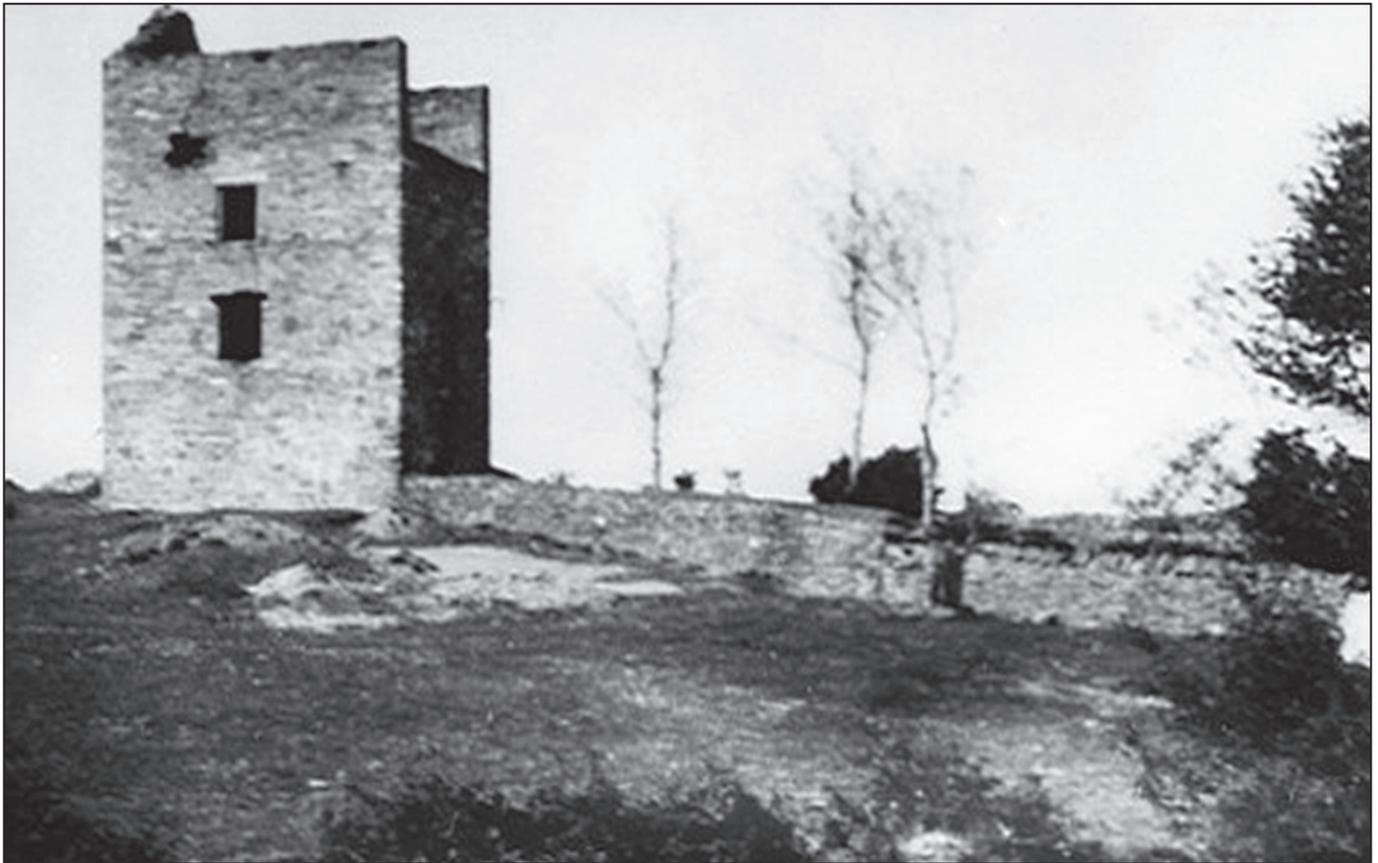
**Figure 9. View of the southern wing wall and the bob wall of the abandoned Creggan Cornish pumping engine house, built to accommodate a 36-inch vertical steam engine. This image is dated 1926, five years before it was demolished. Not even the footprint of the house is visible today. Reproduced by kind permission of the Armagh County Museum**
