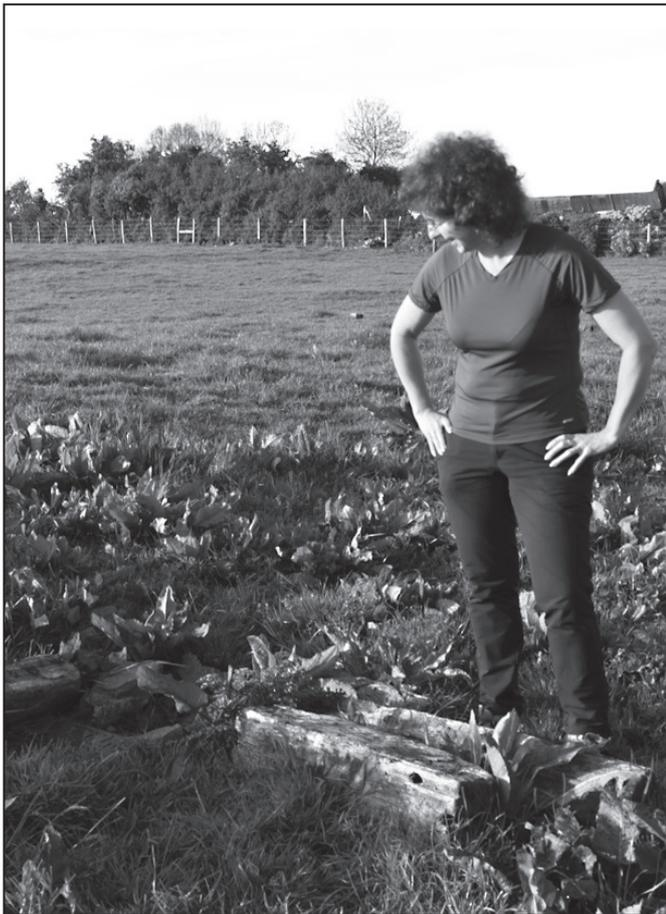
*Figure 14. Sections of pump rod lie close to the manhole cover (just visible far left) of Creggan New Engine Shaft and were probably removed when the shaft was capped in 1995*
