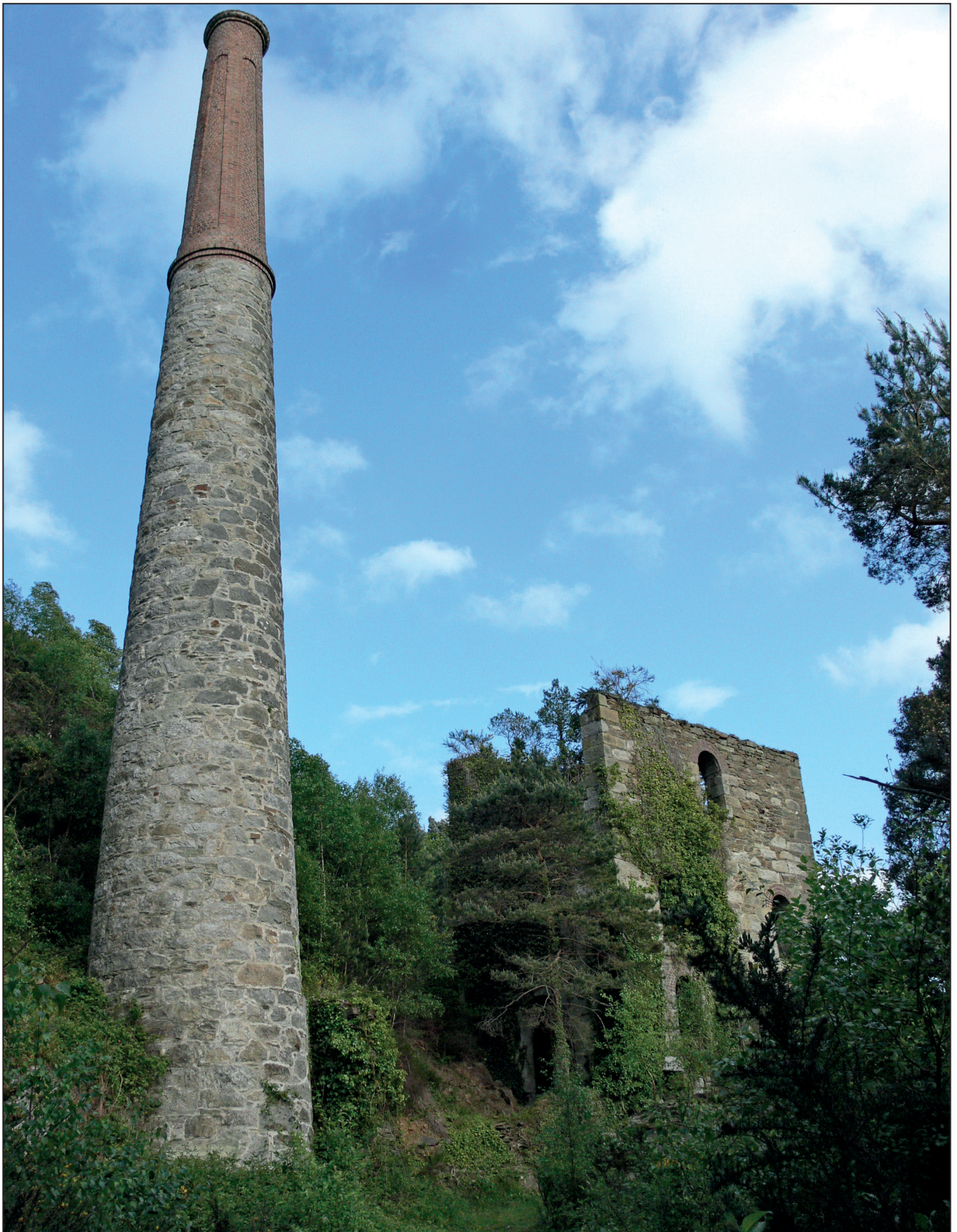
Fig. 13: Williams' Pumping Engine House on the Tigroney Mine, accommodated a 60-inch vertical cylinder steam engine. Built at the Perran Foundry in Cornwall, a concern in which the owners, Messrs Williams, had an interest, this was the largest engine ever erected on an Irish mine. Architecturally significant, having had a back bob and with the walling of its boiler house partially intact, the chimney stack was consolidated in 2003/04, but the remainder of the monument, being colonised by ivy and tree saplings, is in urgent need of consolidation. Image, Martin Critchley, 2007
