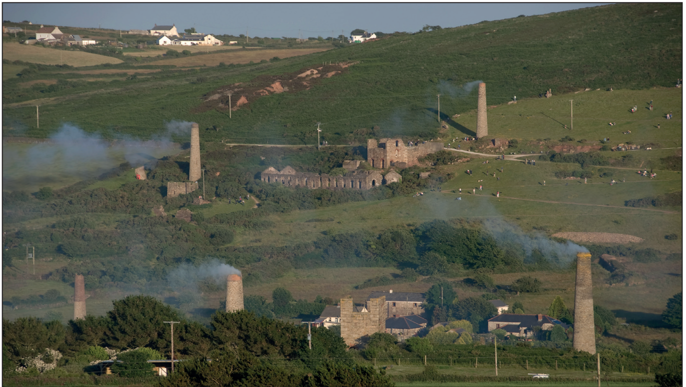
Fig. 3: Consolidated engine houses along the Great Flat Lode at Wheal and West Wheal Basset near Redruth, Cornwall, seen here during the Smoking Chimneys Celebration organised by the Mineral Tramways Heritage Project in 2008. The mine spoil surrounding these monuments was removed when the area was remediated in the 1990s. The works included landscaping, grass seeding and the installation of zig-zag aggregate pathways and picnic tables which did not meet with universal approval. Image, Ainsley Cocks, 2008
