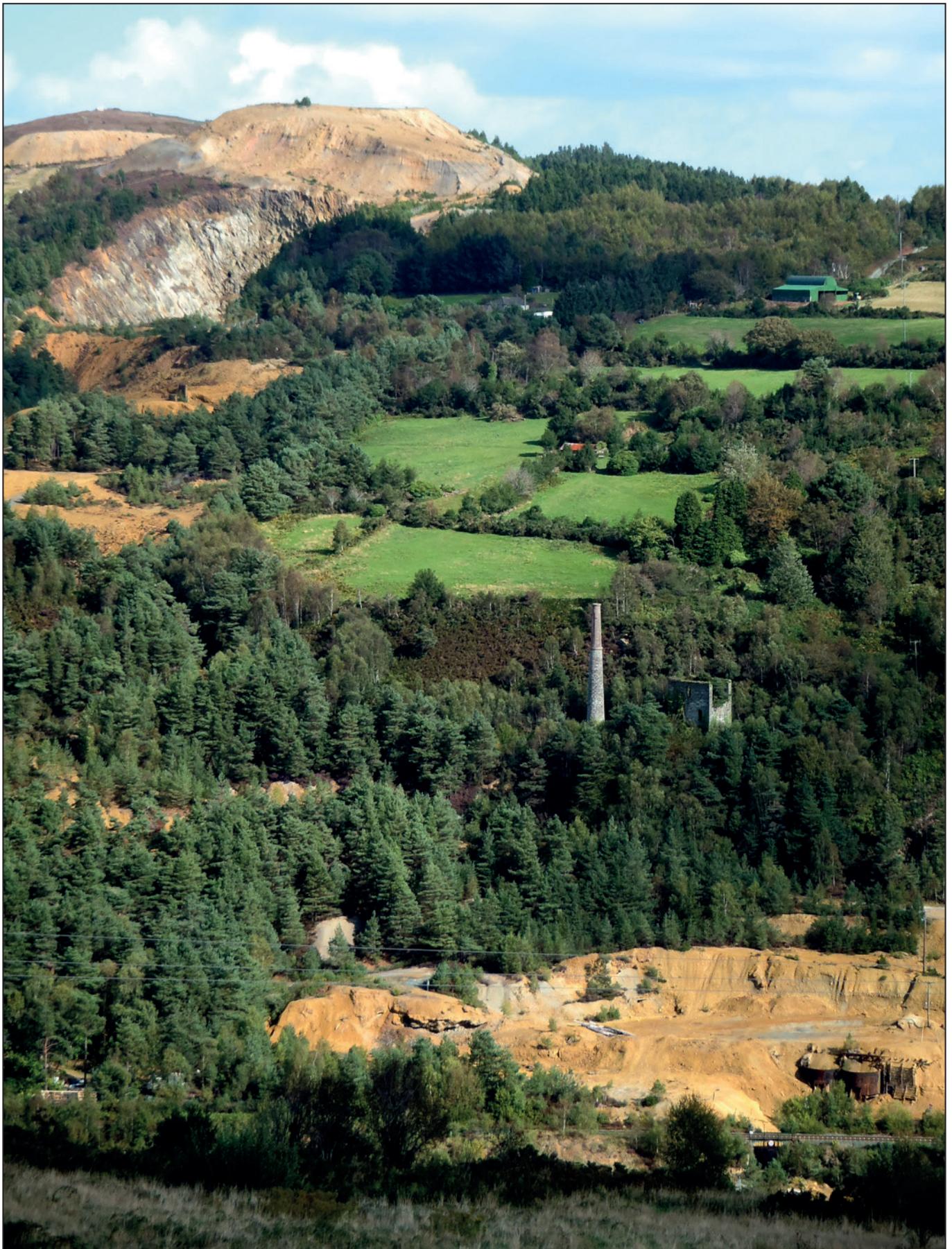
Fig. 15: Some of the discrete elements that together constitute the nationally significant historic mining landscape of East Avoca, can be seen in this image: a nineteenth century Cornish-type engine house; twentieth century ore bins and the concrete base of a crusher; large areas of colourful mine spoil and an open pit that offers an opportunity to view an exposure of volcanogenic sulphide mineralisation. Image, Martin Critchley, 2011
