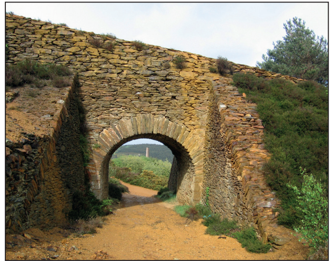
Fig. 12: Drystone tramway arch at Ballymurtagh Mine. Image, Sharron Schwartz, 2007
