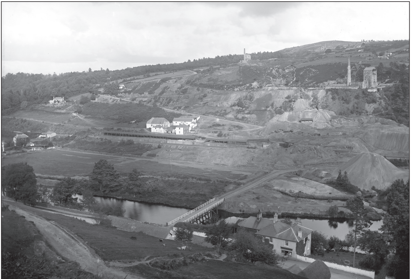
Fig. 1: The rural industrial mining landscape of East Avoca around the turn of the twentieth century, showing extensive spoil heaps and three Cornish-type engine houses on the Tigroney Mine, including the one that accommodated the largest engine ever erected in Ireland (top right). By kind permission of the National Library of Ireland
