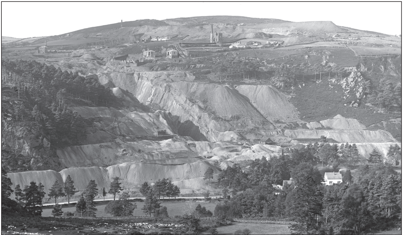
Fig. 2: The West Avoca mines of Ballygahan and Ballymurtagh around the turn of the twentieth century. Note the large open pit (centre), extensive spoil heaps and industrial buildings, including three engine houses. The open pit, expanded in the mid twentieth century, has since been used as an unlined landfill (see Fig. 22) and the majority of the surface landscaped and grassed over. The loss of the remaining spoil (top right), would further seriously degrade what remains of this historic mining landscape. By kind permission of the National Library of Ireland
