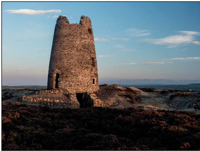
Fig. 9: The consolidated windmill at Parys Mountain Mine now serves as a shelter for walkers and houses several interpretation boards. This is one of only two windmills to survive on a metal mine site in Britain or Ireland, the other being at the Newtownards Mine near Belfast in Northern Ireland. Photograph, Sharron Schwartz, 2013
