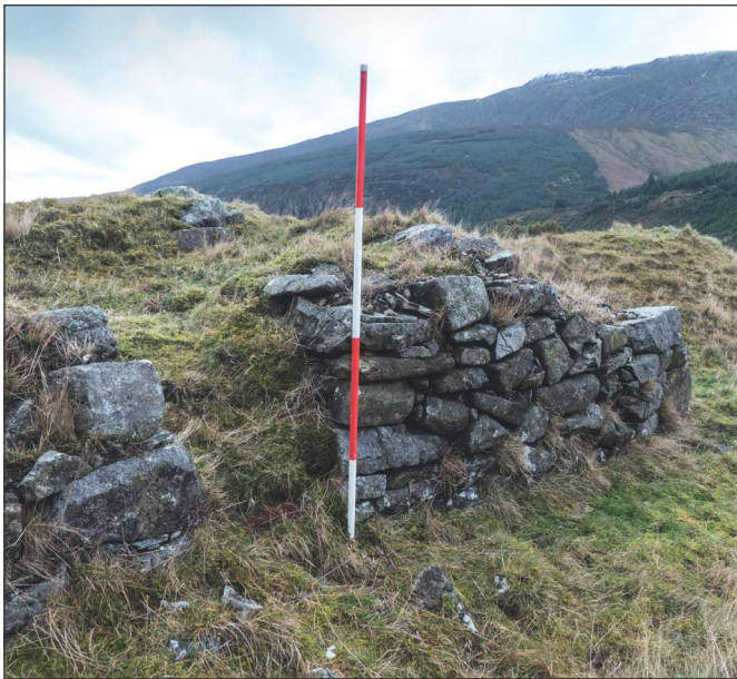
Fig. 24 left and Fig. 25 right, depict the small dressing floor constructed of random moorstone boulders close to the entrance of Adit Four. Built on the orders of Captain Griffith in 1853, this, and another less well-defined dressing floor at Shallow Adit, were meant to be only a temporary measure before purpose built dressing floors were constructed at Deep Adit. The lodestuff was washed, sorted and crudely reduced at this small dressing area before being transported to the valley floor. The 'V'-shaped notch in the wall of Fig. 24 is where a picking grate was likely positioned, fed by water from the adit. One can only imagine how brutal it would have been to work in such an elevated, exposed place
