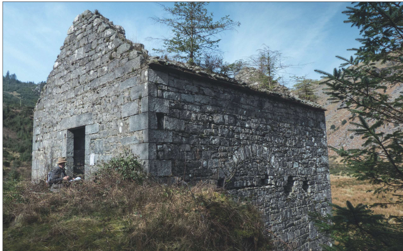
Fig. 35: The rear of the crusher house featuring the doorway into the upper storey where the ore was fed into a hopper. Note the joist pocket in the eastern wall at the level of the rear doorway that probably held a timber supporting either the waterwheel frame or a launder bringing water onto the wheel
