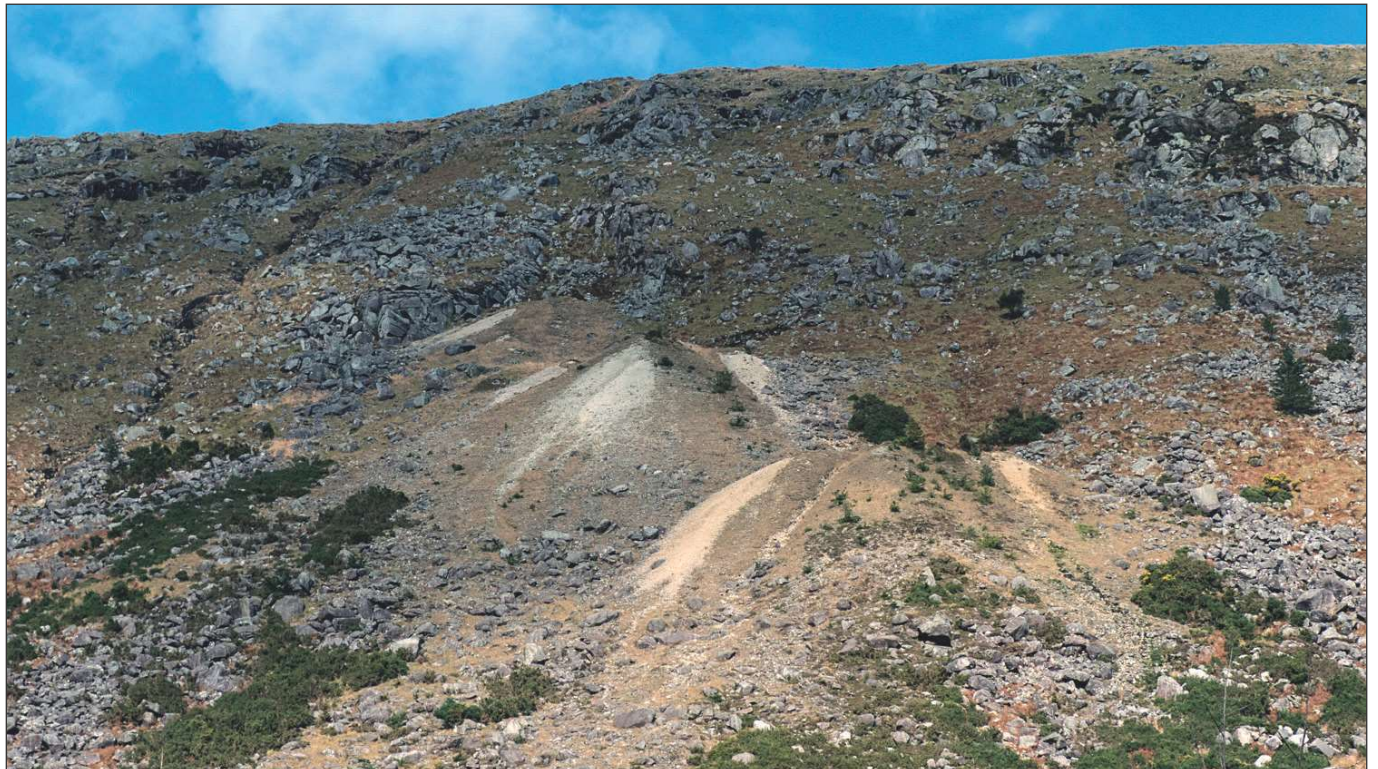
Fig. 23: The Ballygoneen Mine, sited high in the cliffs at the head of Glenmalure seen here from the Stony Road that runs through the valley from Rathdrum over the Wicklow Mountains to the Glen of Imaal. Three of the mine's five levels are betrayed by spoil heaps. Adit Four (centre) has a well-defined crude dressing area sited close to its portal
