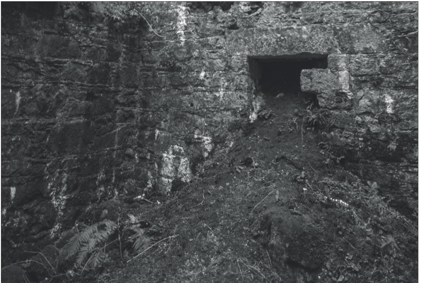
Fig. 38: Opening in the rear interior wall of the crusher house which appears to be a blocked up doorway, the masonry infill of which has failed
