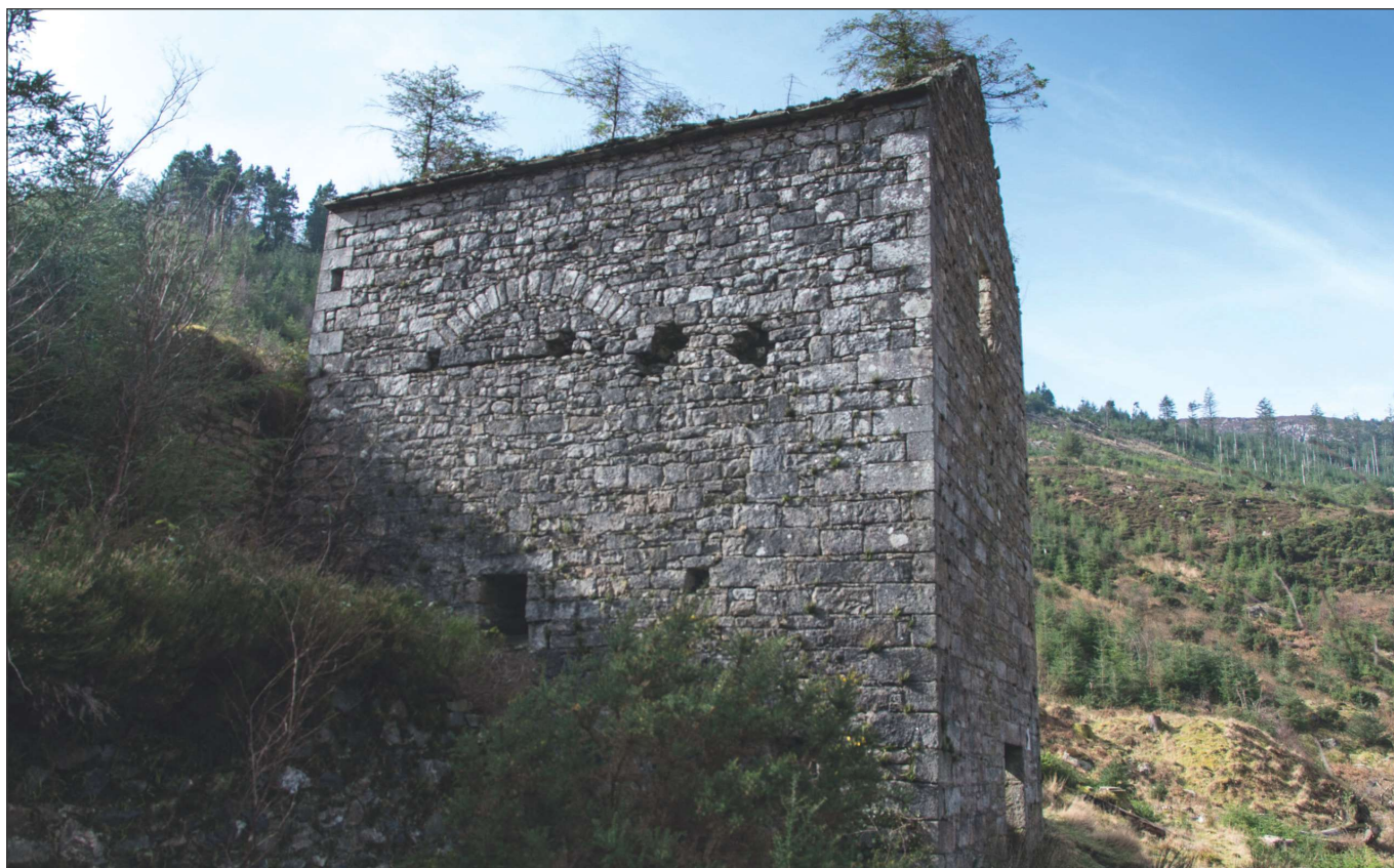
Fig. 34: Eastern wall of the New Crusher House. Note the discharging arch built above the square aperture which accommodated the drive shaft that transferred power from the waterwheel to operate the crushing rolls inside the building
