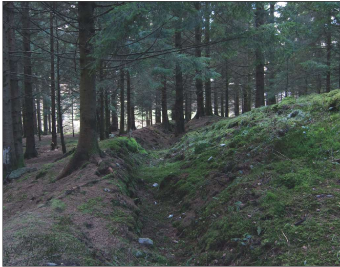
Fig. 20: Leat channel that conveyed water to the Glenmalure Mine dressing floors contouring round the back of a small knoll before meeting Mill Brook
