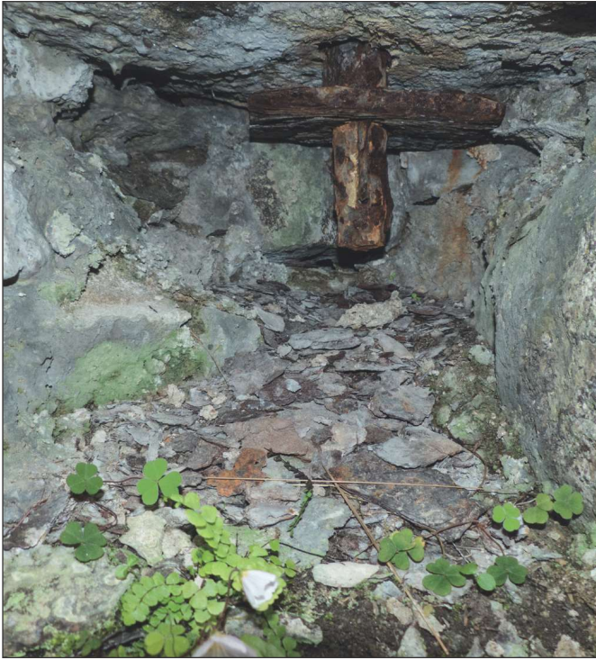
Fig. 30: View inside a 'crow-hole' at the bottom of the waterwheel casement. Used during the installation of the machinery, 'crow-holes' were vital access points for attaching a plate and fixing cotter on the end an iron bolt that secured an item of machinery above. Only the plate is depicted here
