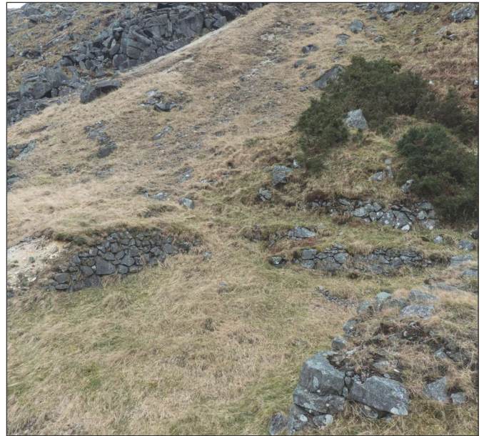
Fig. 24 left and Fig. 25 right, depict the small dressing floor constructed of random moorstone boulders close to the entrance of Adit Four. Built on the orders of Captain Griffith in 1853, this, and another less well-defined dressing floor at Shallow Adit, were meant to be only a temporary measure before purpose built dressing floors were constructed at Deep Adit. The lodestuff was washed, sorted and crudely reduced at this small dressing area before being transported to the valley floor. The 'V'-shaped notch in the wall of Fig. 24 is where a picking grate was likely positioned, fed by water from the adit. One can only imagine how brutal it would have been to work in such an elevated, exposed place
