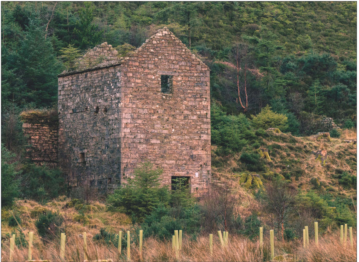
Fig. 33: The New Crusher House at the Baravore Mine, a well-constructed building erected in 1859-60 to accommodate what we believe to have been a multiple rolls crusher and is the finest extant example of a such a crusher house in Ireland. Yet, despite its solid appearance, urgent conservation work is required to ensure it does not suffer a similar fate as the Old Crusher House, the front wall of which experienced a significant collapse in the spring of 2013
