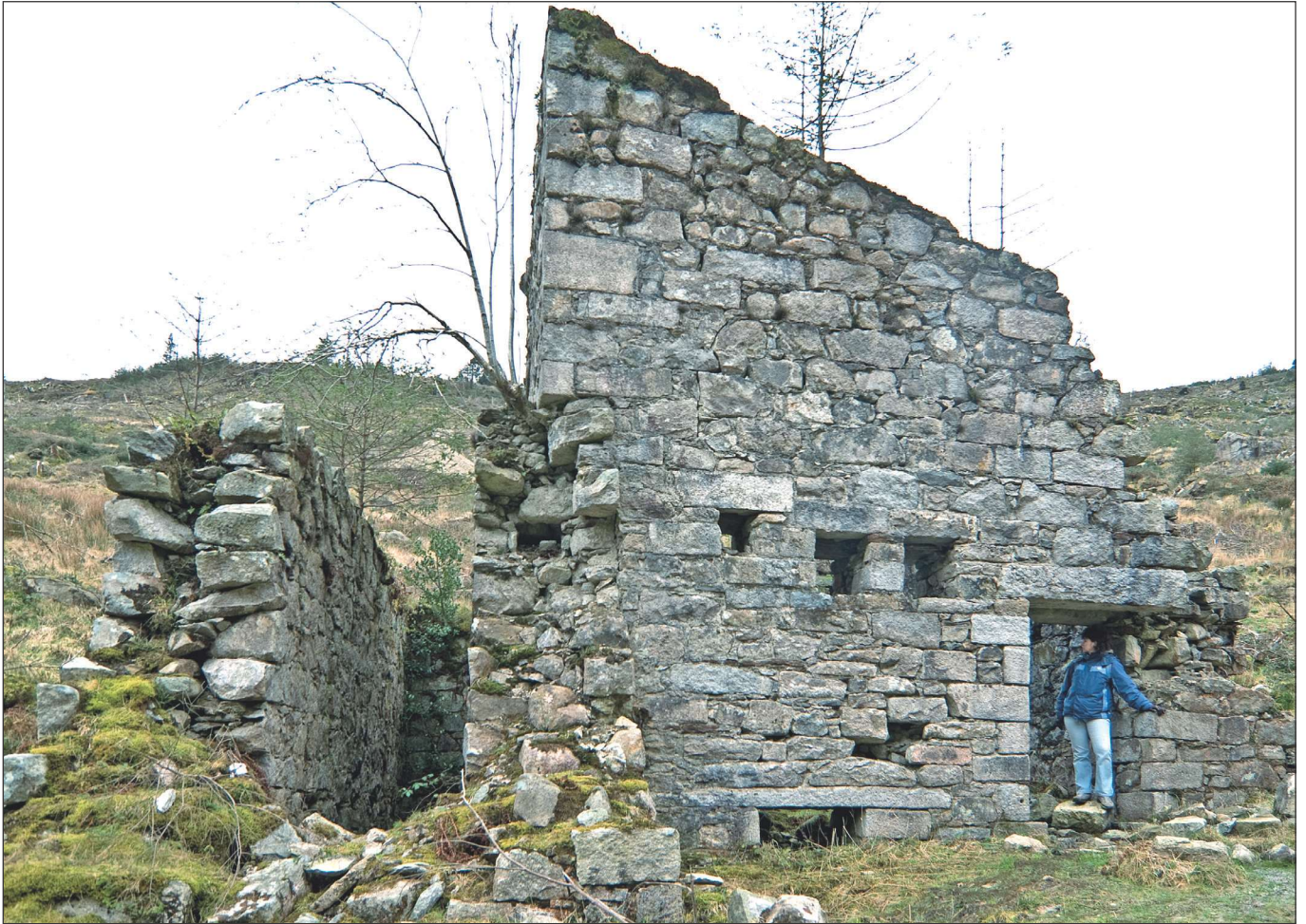
Fig. 26: The Old Crusher House and waterwheel casement for a single set of Cornish rolls at Baravore Mine, pictured in March 2008 before part of its front wall collapsed in late winter, 2013 (see Fig. 27 below). This mid-nineteenth century building, listed in the Record of Protected Structures for County Wicklow, is the finest industrial monument of its type in Ireland. Its preservation is a matter of urgency
