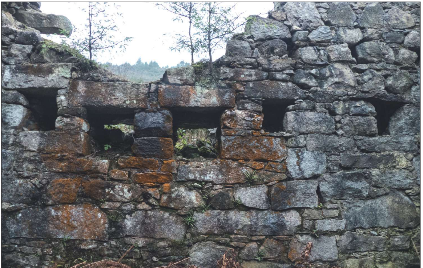
Fig. 31: Interior rear wall of the crusher house showing joist pockets for support timbers relating to (L-R) the Raff-wheel; the Cornish rolls (parallel larger apertures); the trommel and axle bearing. These joist pockets are repeated in the front wall of the crusher house
