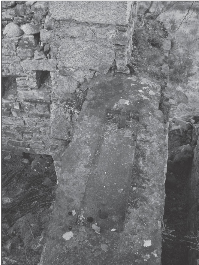
Fig. 28 (left): The axle mounting plate with two protruding 'bolts'. These run the length of the crusher house wall as depicted in Fig. 29 (right) and emerge in two 'crow holes' at the base of the waterwheel casement (Fig. 30)
